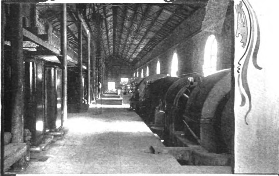
Interior of Powerhouse
